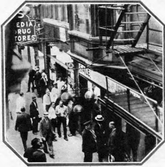
The scene of one of the Jersey Kid's cleverest jobs—a loan office at 5146 Market Street, Philadelphia. The loot: sixty grand
