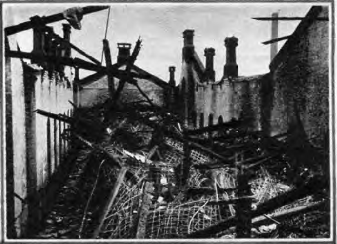
Where Death arrived! The unfinished and unoccupied cell block, where the conflagration had its origin
